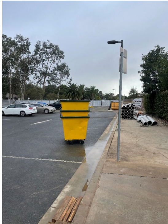
Photo 2 – Skip bins, storage and construction parking area
