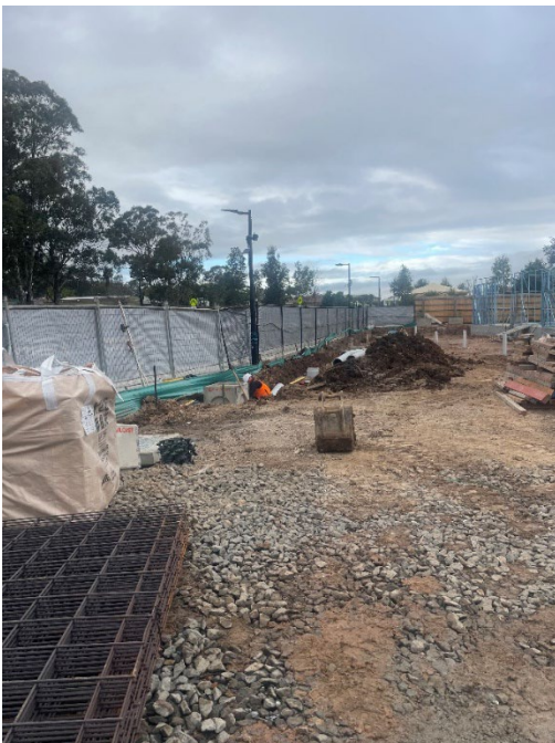
Photo 3 – fencing and sediment fence
