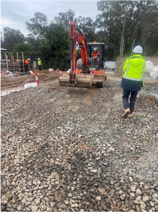
Photo 1 – Showing ballast to prevent mud tracking
